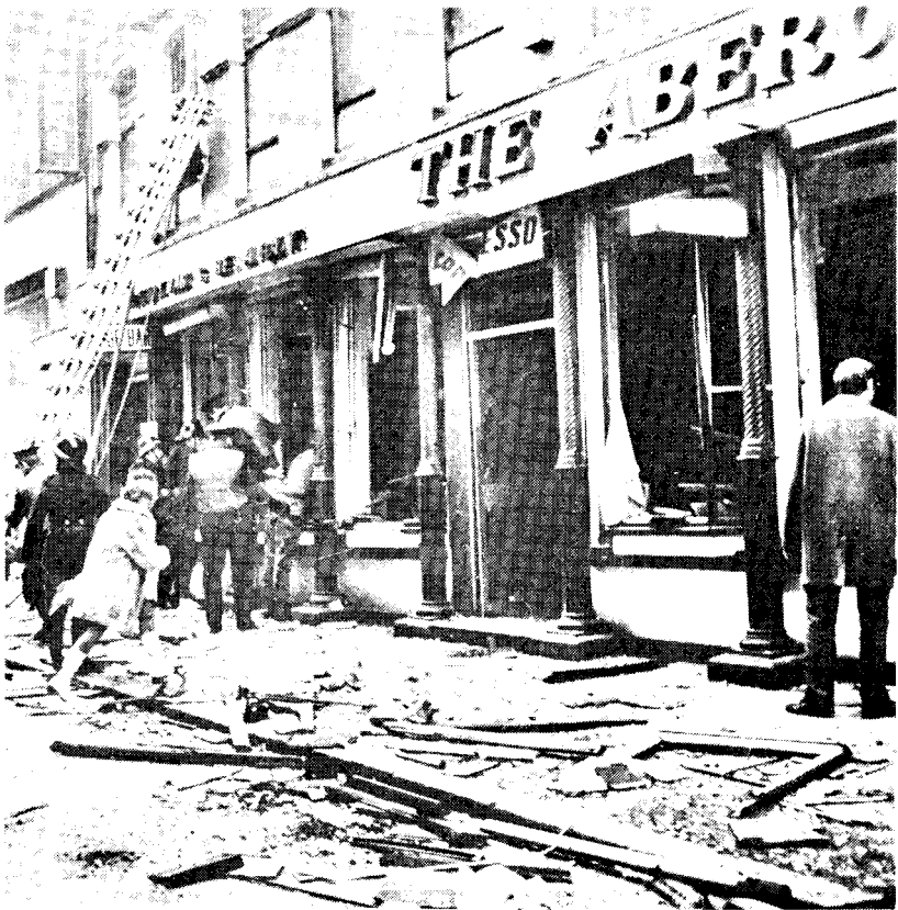
The Abercorn: a Restaurant crowded with shoppers having their afternoon tea, then it was a scene of death and destruction wrecked by another I.R.A. bomb
