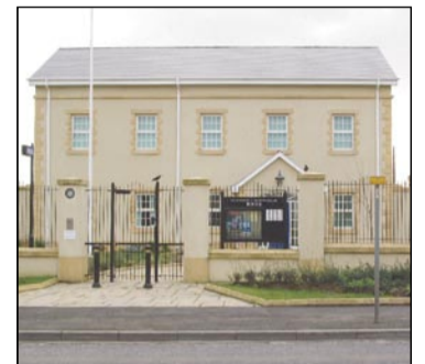
Moirra PSNI Station - setting new standards in design.
