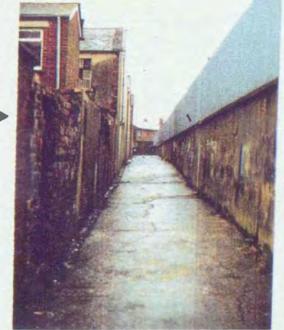
▶ SERVICE ALLEY TO REARS OF 40 - 68 OLDPARK AVENUE TOWARDS OLDPARK ROAD SIDE
