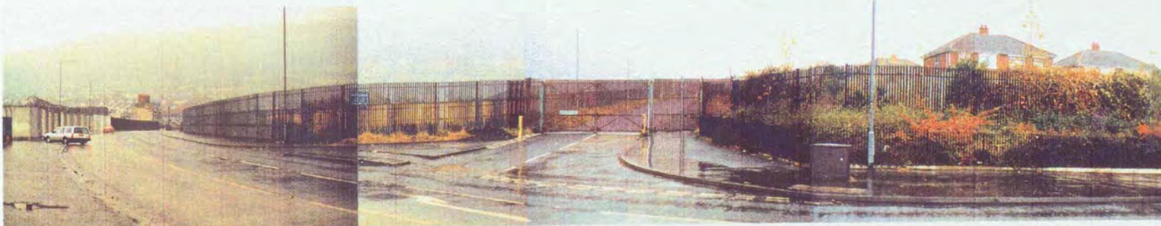
▲ SECOND GATE AND FRONTAGE ARRANGEMENT FROM SPRINGFIELD ROAD
