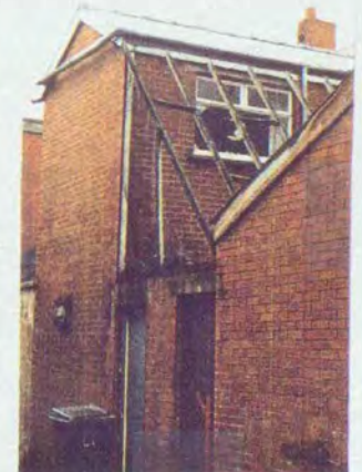
MAKESHIFT PROTECTORS ERECTED BY N.I.H.E.
