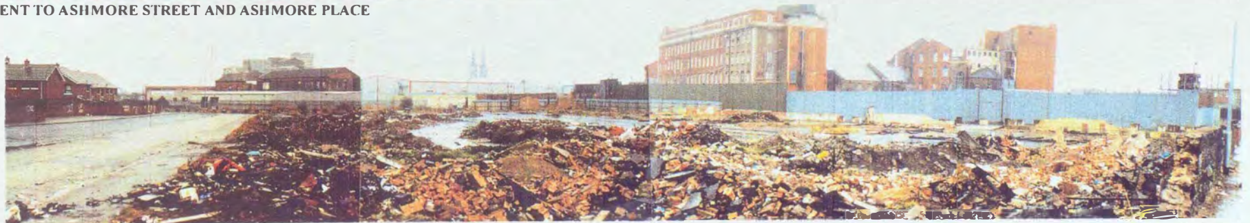
▲ VIEW OVER FORMER F.G. WILSON SITE AND OLD MILL BUILDINGS
