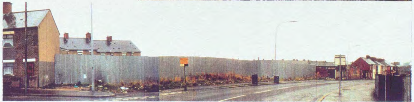
▲ NO 1 TORRENS AVENUE ALONG OLDPARK ROAD FRONTAGE
