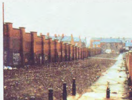
▲ UNMADE GROUND TO 168 AND 170 CLIFTONVILLE ROAD
