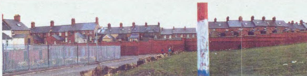
▲ FROM TORRENS CRESCENT OVER DIVIDE TO BACKS OF HOUSING ON OLDPARK AVENUE
